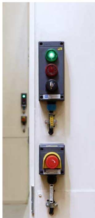
ATEX key switch open-close ATEX emergency stop mushroom-type push-button
